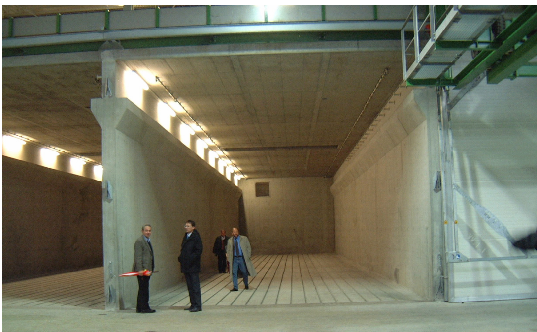
Figure 18 Example of a rotting box for the principal rotting of heavy fraction from MSW
